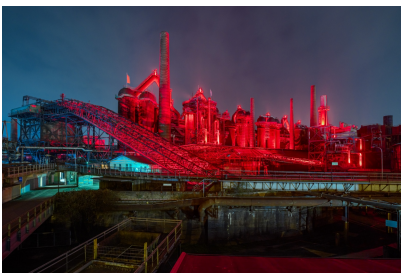
The World Heritage Site Völklinger Hütte by night
